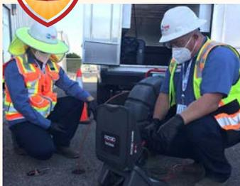
Natural gas utilities across the country have discovered locations where natural gas pipes were inadvertently installed through sewer pipes.
